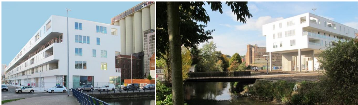
Figure 5: Pictures of the north side (left) and south side (right) of the 'Balk van Beel'
